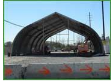
Fabric structures are built over contaminated areas at MGP sites.
